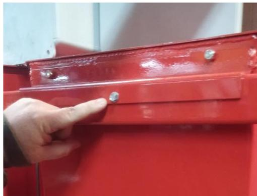
12. Attach the Game Clock Display Box from Support Beam #3 using provided nuts, washers, and bolts.
